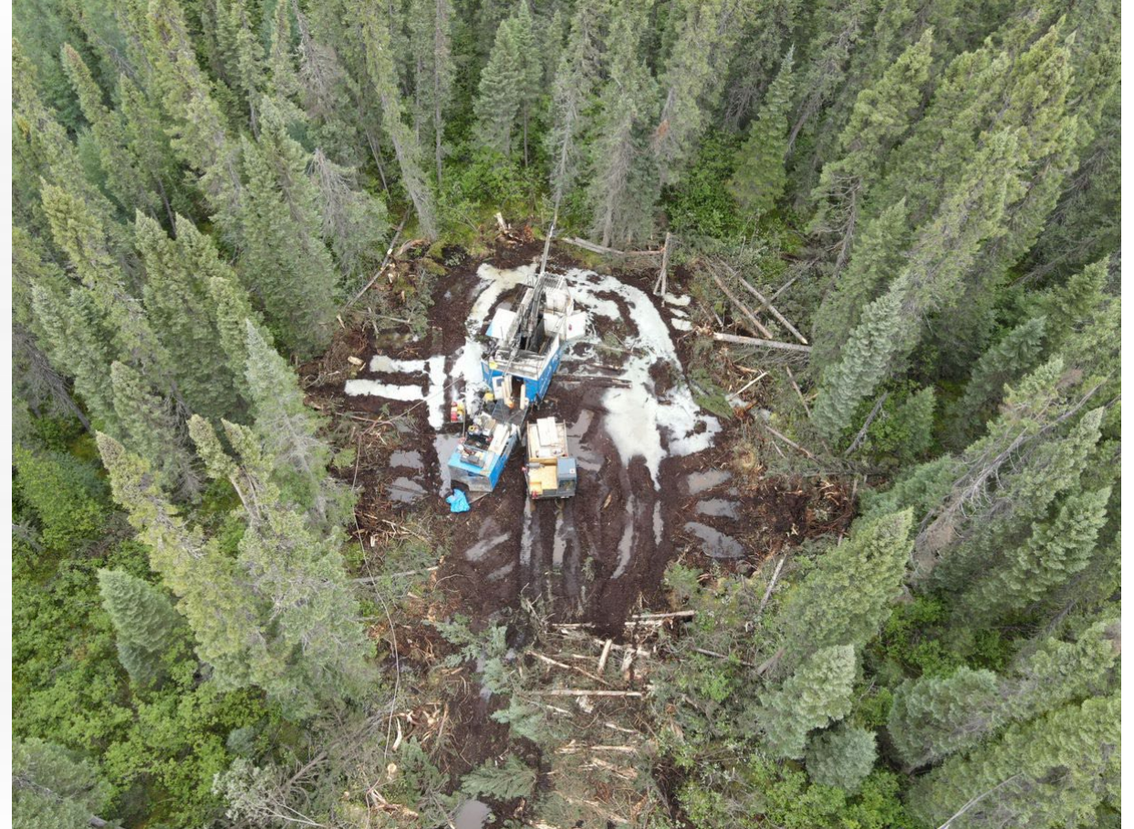
Drilling at Thierry
